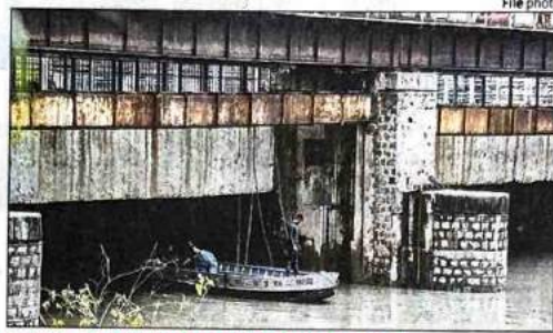
HOPING TO AVOID A REPEAT AT ITO BARRAGE
