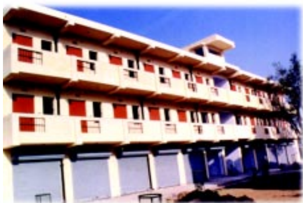
Flats and shops constructed under Garhia Lohar Resettlement Project in Mangolpuri
