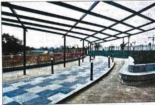
Walkway along a drain inaugurated on Tuesday. VIPIN KUMAR/HT
